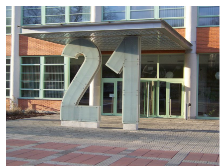
Detail of the building entrance
